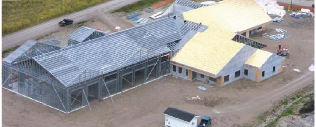
It was a race against time to build the facility to a closed-in state in one construction season – including the pouring of a 2,323m<sup>2</sup> (25,000 sq. ft.) engineered concrete slab. As well, fabrication and erection needed to be as simple as possible given the lack of a local highly-skilled labour force.
