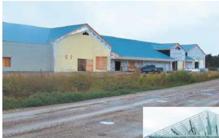
Precut material and components, were assembled over the course of the winter months in Moose Factory. Construction on site started in the spring. Wall panels were shipped to the site in July and assembly of the superstructure took place in July and August.
