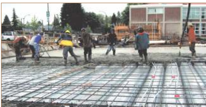
Fast Track Construction Accommodates duct work, conduit and other building services
