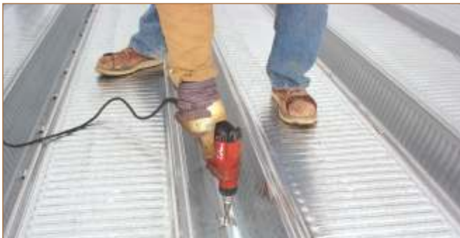
Rigid Steel Deck Provides safe unshored work platform
