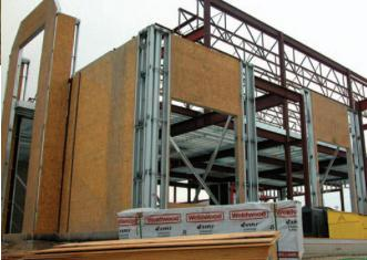
Many of the fire concerns were classified as non-combustible with the switch to light steel framing. This is of course an advantage where insurance rates are concerned.
