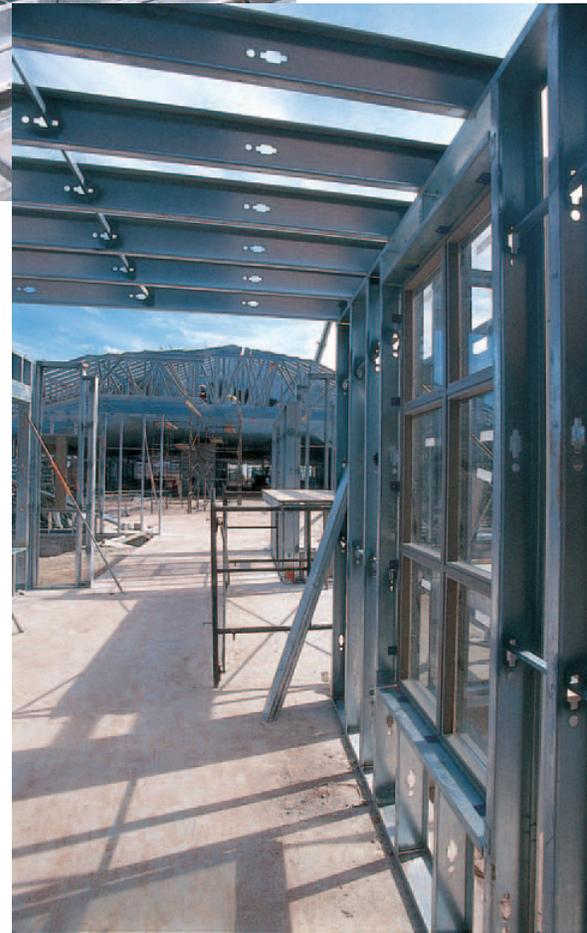
Genesis steel wall panels are used for The Clubhouse walls, as well as for the ground-level links to the residential blocks. LSF sections were used for these wall panels.
