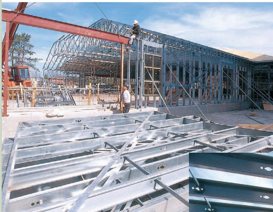
Genesis™ steel roof trusses and wall panels made from light steel framing contributed significantly to meeting several of the prime considerations - light weight, noncombustibility and speed of erection.
